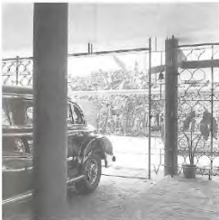
Car park looks towards entrance showing the "flat" slab without beams
