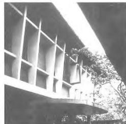
Detail of sunbreakers to bedrooms.
